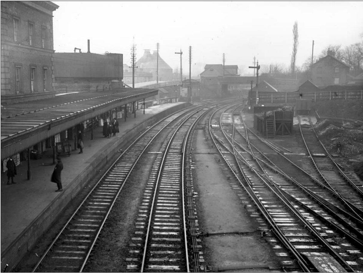
Photo 2.14 Bishops Stortford station. Outside slip on the right which forms part of an asymmetrical cross-over. (NRM Windwood Collection GE176).
