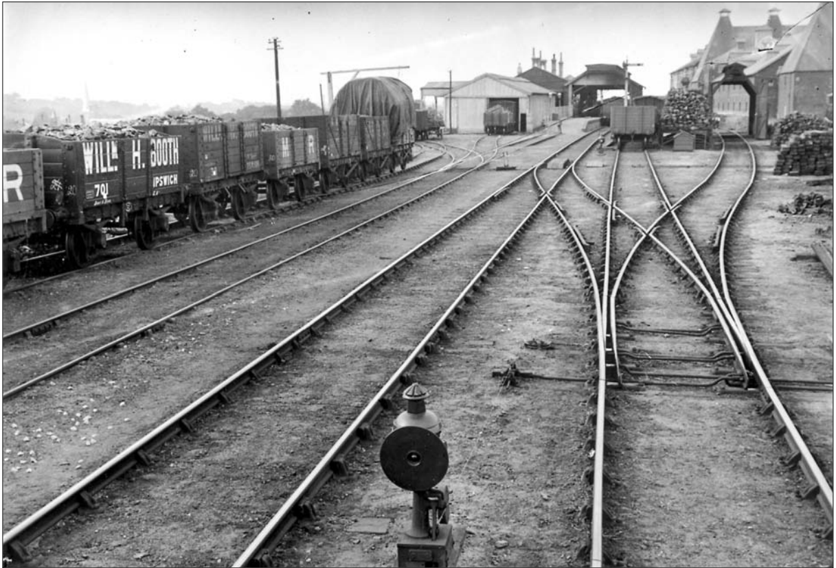
Photo 2.3 Symmetrical three throw turnout in Hadleigh goods yard. A second asymmetrical three throw is just visible in the top centre of the photo. (NRM Windwood Collection GE1043)
