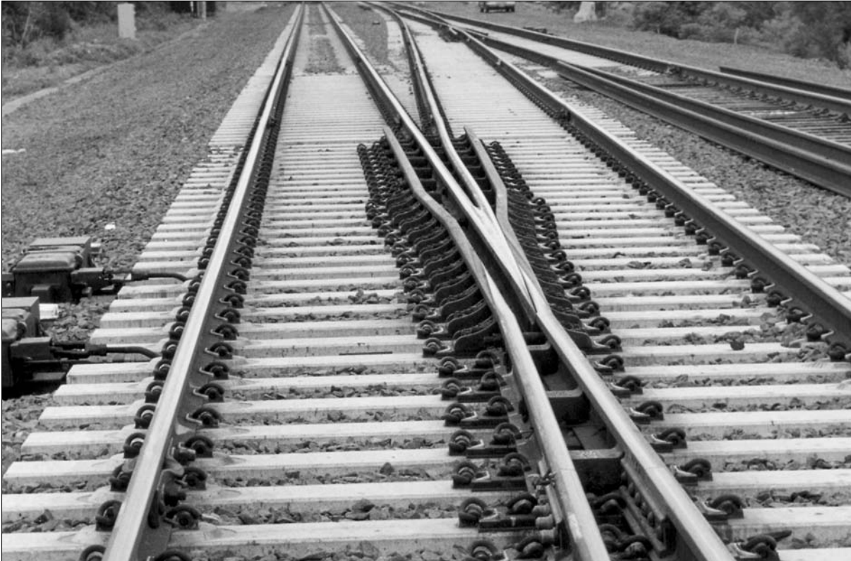
Photo 2.8 Swing nose crossing. Note the absence of check rails. A suitable prototype for multi-standard pointwork for model railway test tracks. (Pandrol Rail Fastenings Ltd).
