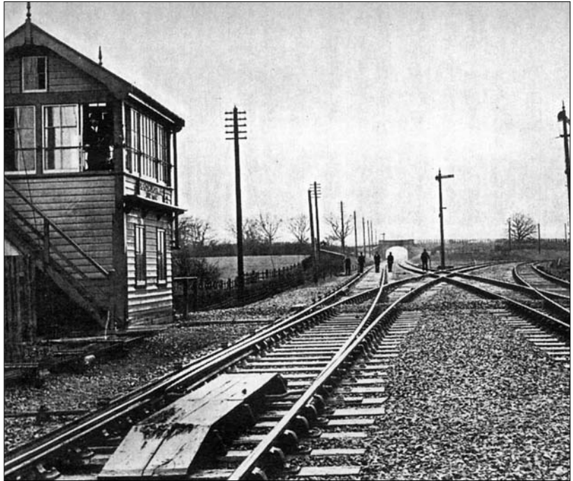
Photo 2.10 High speed double junction at Grendon Underwood, G.C.R., with diamond set at 1 in 8. (Loco Publishing Co).
