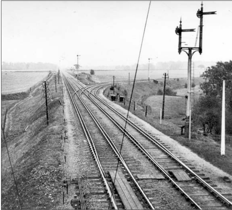
Photo 2.19 Interlaced turnouts at Wymondham Junction with the Focsett Branch. (HMRS Collection).
