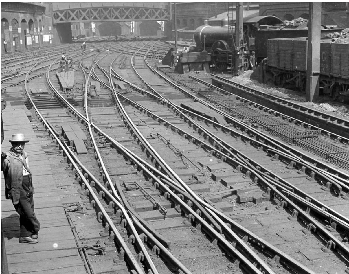
Photo 2.12 Trackwork at Liverpool Street showing two single slips in the foreground leading to a double slip in the middle distance. The presence of continuous check rails in the left hand roads suggests that the curves are less than 10 chains radius. (NRM Windwood Collection GE868).
