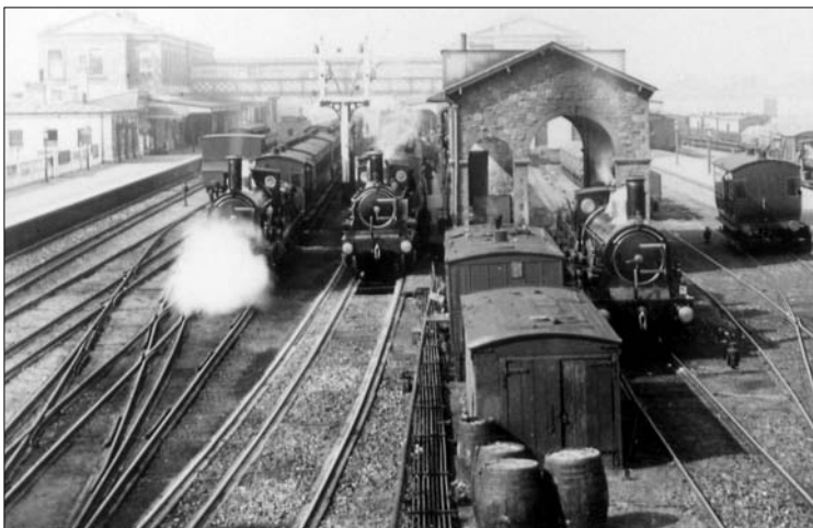
Photo 2.20 A mixed gauge crossover. Because the common rail is required to be on the outside adjacent to the platform face, the narrow gauge line has to side step to attain the correct alignment. Careful use of guide rails allow this to be achieved without using additional moving blades. (HMRS Collection).
