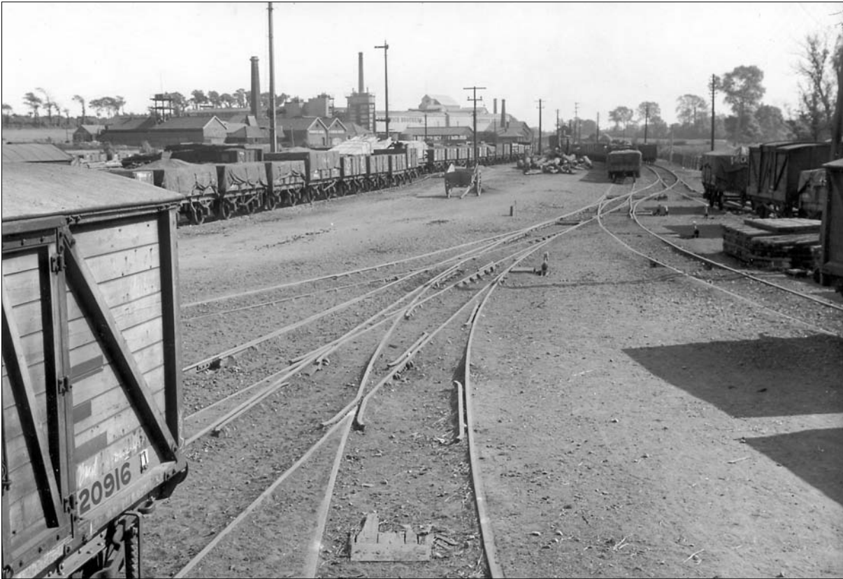
Photo 2.2 A double tandem turnout leading off from a double slip at Stowmarket Goods Yard. (NRM Windwood Collection GE1005)
